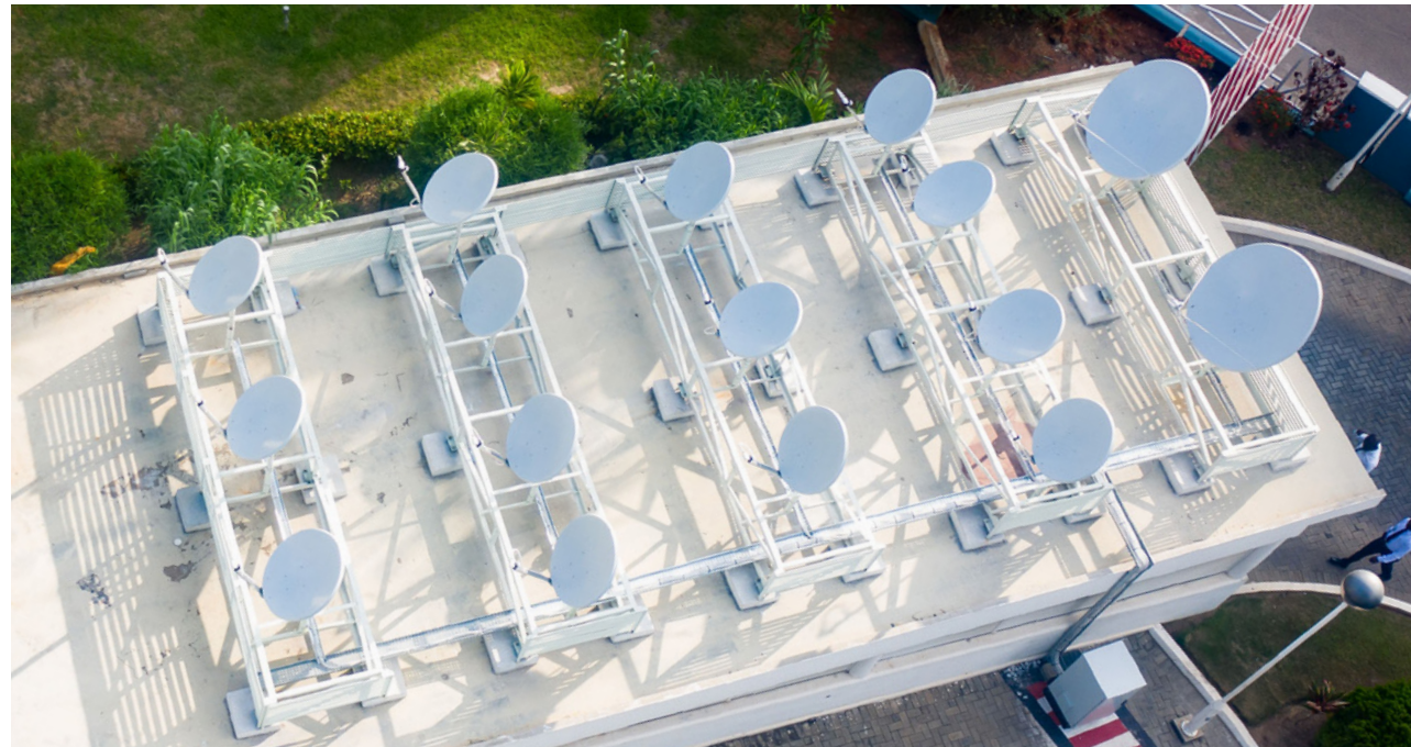
Aerial view of Terrestrial and Satellite Receiving Antennae
