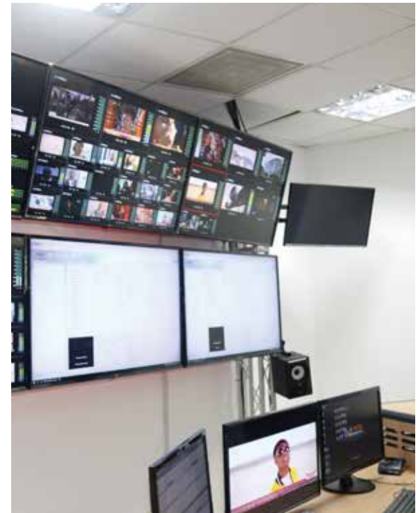
The Broadcast Monitoring Centre where Engineers have a real-time overview of the technical output of authorised TV and FM stations
