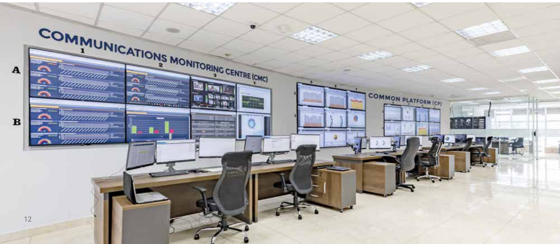
The Network Monitoring Centre sits in the Communications Monitoring Centre
